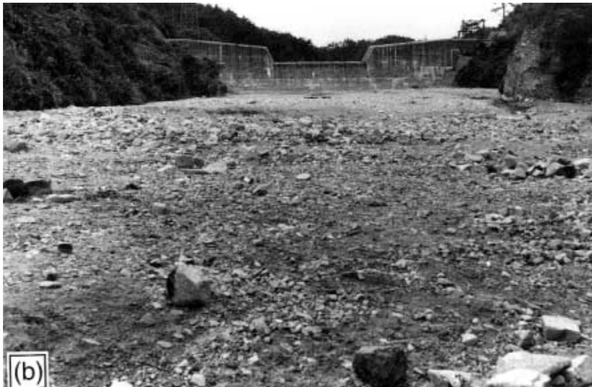
Figure 33. Check dam in Hyogo, Japan (30 m high, 78 m long, storage capacity 300,000 m<sup>3</sup>), (a) before and (b) after a debris flow. (Photo from United Nations, 1996)
