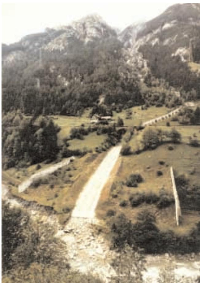
**Figure 32. Steel-cell barrage structure set up on the Issyk River, Kazakhstan. (Photo from United Nations, 1996)**
